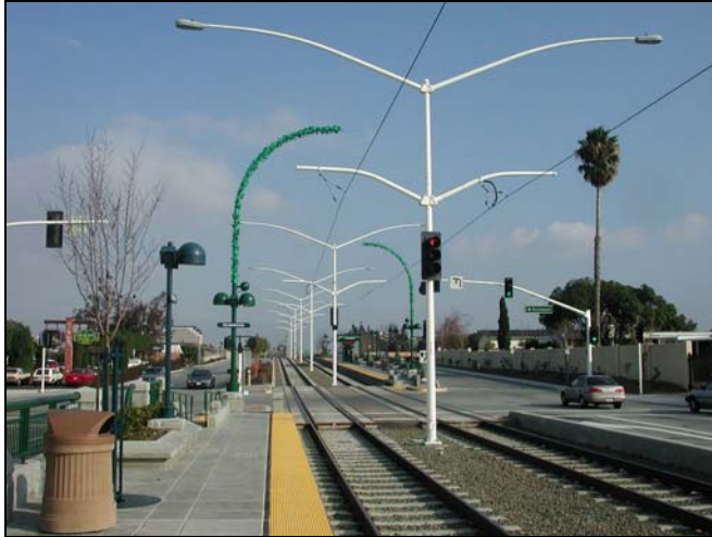
Fig. 2 - Joint-use Center Cantilevered Supports (San Jose, CA)
