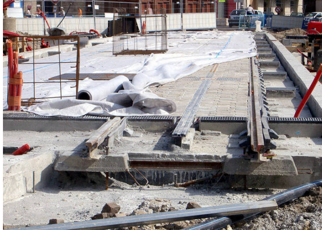
Fig. 15 - Installation of APS System
