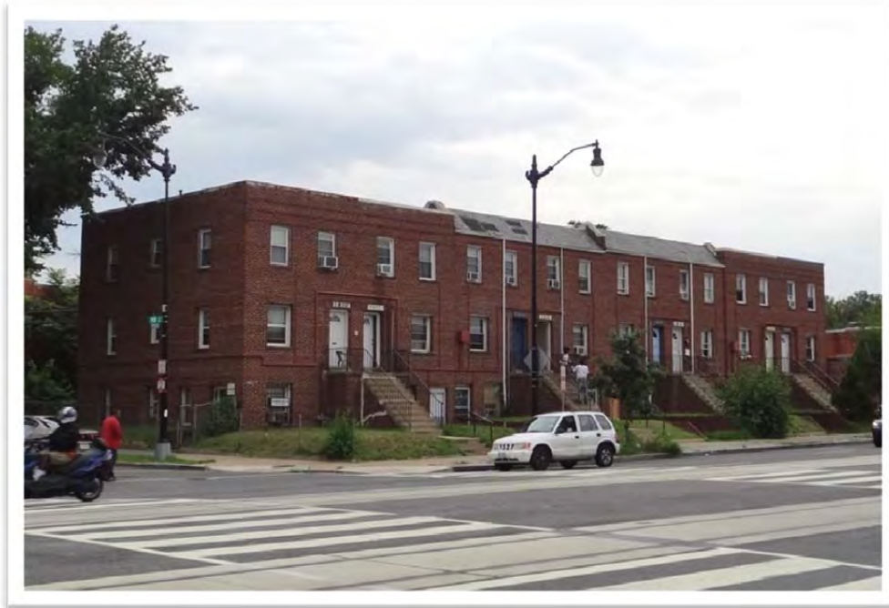
Figure 29 | 1800-1814 Benning Road NE, view northeast (HDR 2012)
