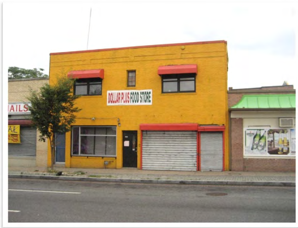
Figure 30 | 1822-1826 Benning Road NE, view north (HDR 2012)
