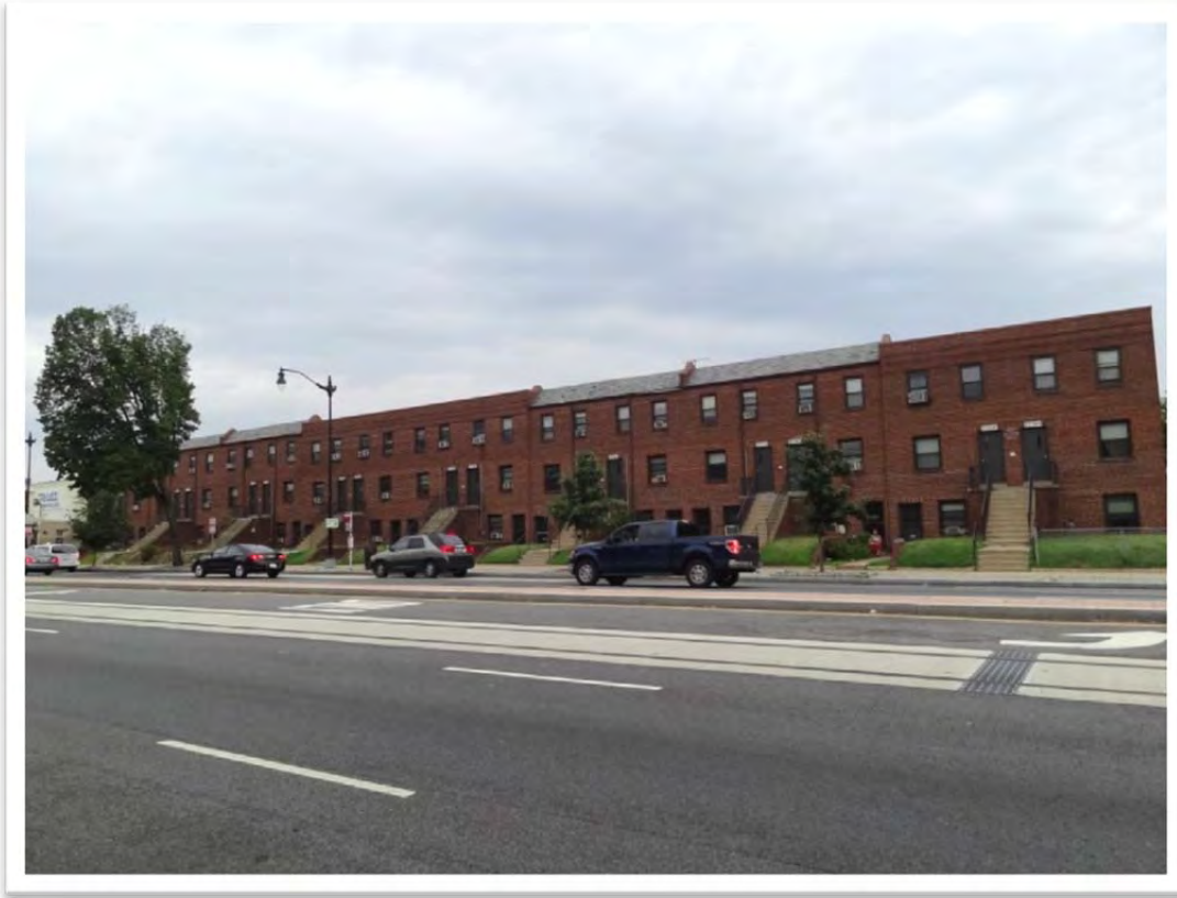
Figure 23 | 1720-1748 Benning Road NE, view northwest (HDR 2012)
