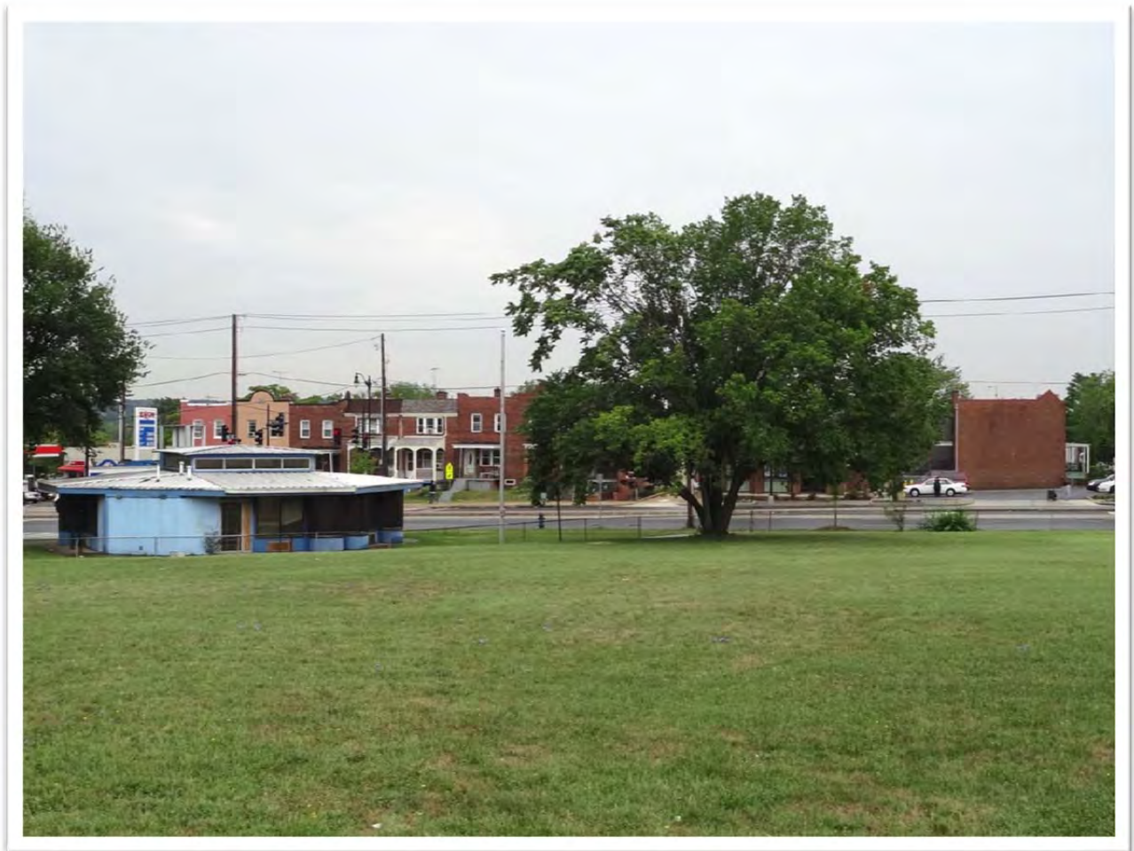
Figure 41 | View south of overhead wires along Benning Road, south of the school campus (HDR 2012)
