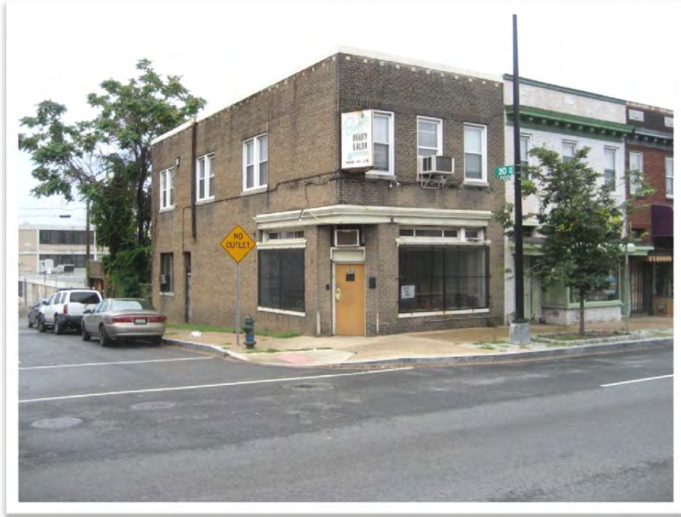
Figure 31 | 1923 Benning Road NE, view southwest (HDR 2012)
