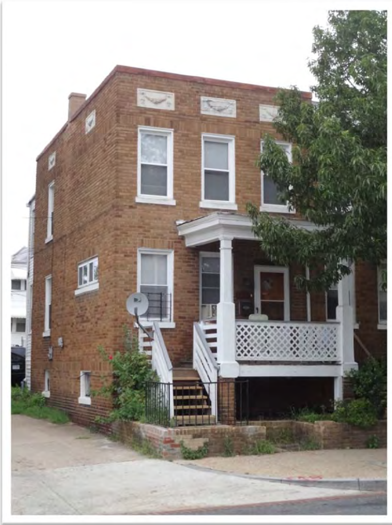
Figure 22 | 1910 Benning Road NE, view northeast (HDR 2012)
