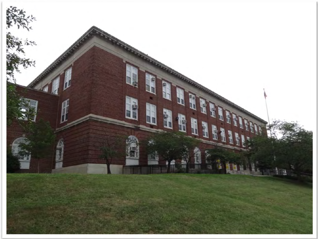
Figure 36 | Browne Junior High School, view northwest (HDR 2012)
