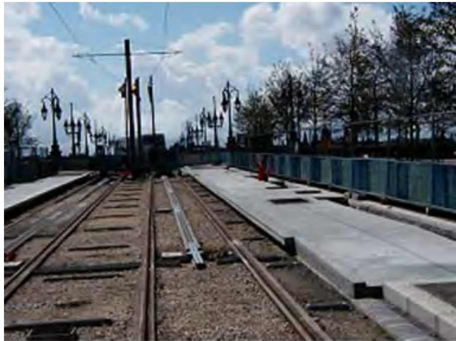
Station Transition Point
