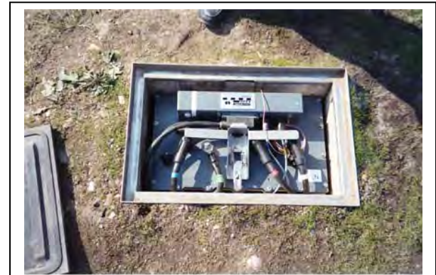
INSTALLED POWER RAIL CONTROL UNIT
