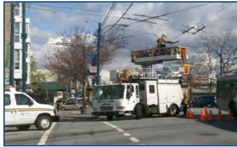
Overhead wire maintenance
