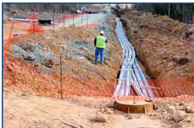
Duct bank construction
