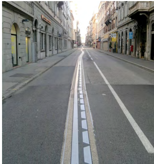
View of a Stream power rail on via Mizzoni, Trieste (© L. Fascia)
